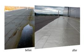
For our important client, the CTP group, it was necessary to carry out roof renovation on an administrative building which was damaged, poorly sealed and leaked in an area which was connected to a neighbouring storage facility. Due to these defects there was a leak into the building which was in danger of damaging it.
